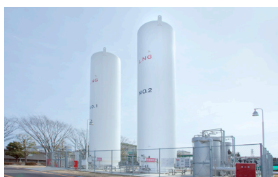
LNG satellite facility and small boiler facility
