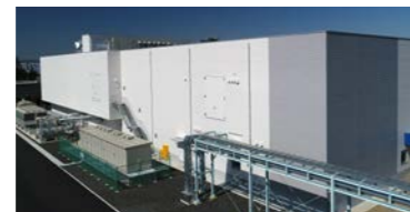
Newly constructed Ashikaga injection drug manufacturing building for high-potency drugs (anticancer drugs, etc.)
