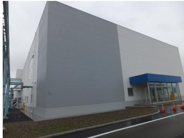
New injection building (Ashikaga)
