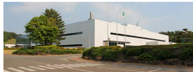
Nishine Plant exterior
