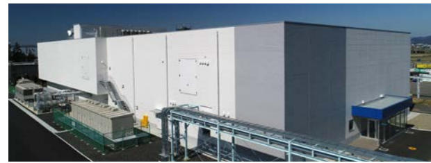
Newly constructed Ashikaga injection drug manufacturing building for high-potency drugs (anticancer drugs, etc.)
